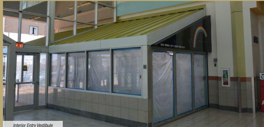
Interior Entry Vestibule
